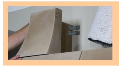
The overhood stones are fastened to the wall with Lbrackets.
