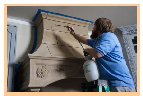
The stones must be saturated with water before grouting. This prevents the white cement from leaching into the stones. Once grouted the stones might take 2-3 weeks to dry. If the stones become chalking after 2-3 weeks then you may want to apply an acid wash to remove this film.
