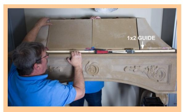
A 1x2 guide is used to help support the bottom row of the overhood.
