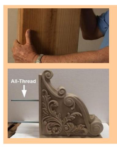
Additional backing in the wall will be required. (2) 2x12 studs stacked back to back must be added behind the location of the corbels and header return.
