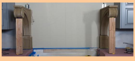
Then a 2x4 support is placed for the remainder of the installation.
