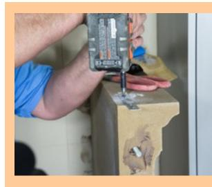
Brick ties are attached from the top as well as additional epoxy and corner brackets used on the inside.
